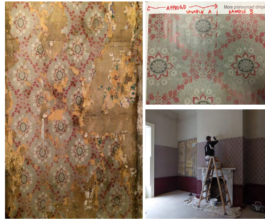
Figs 6.7: Conservation and restoration works which involve preserving surviving fragments of wallpaper and restoring missing sections with new, matching paper.
