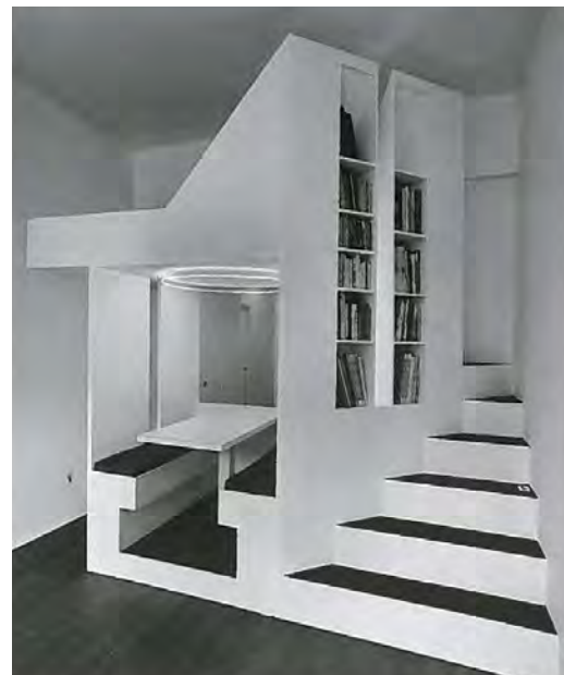
Figs 6.10 : Installation of a new habitable structure inside an existing historic volume
