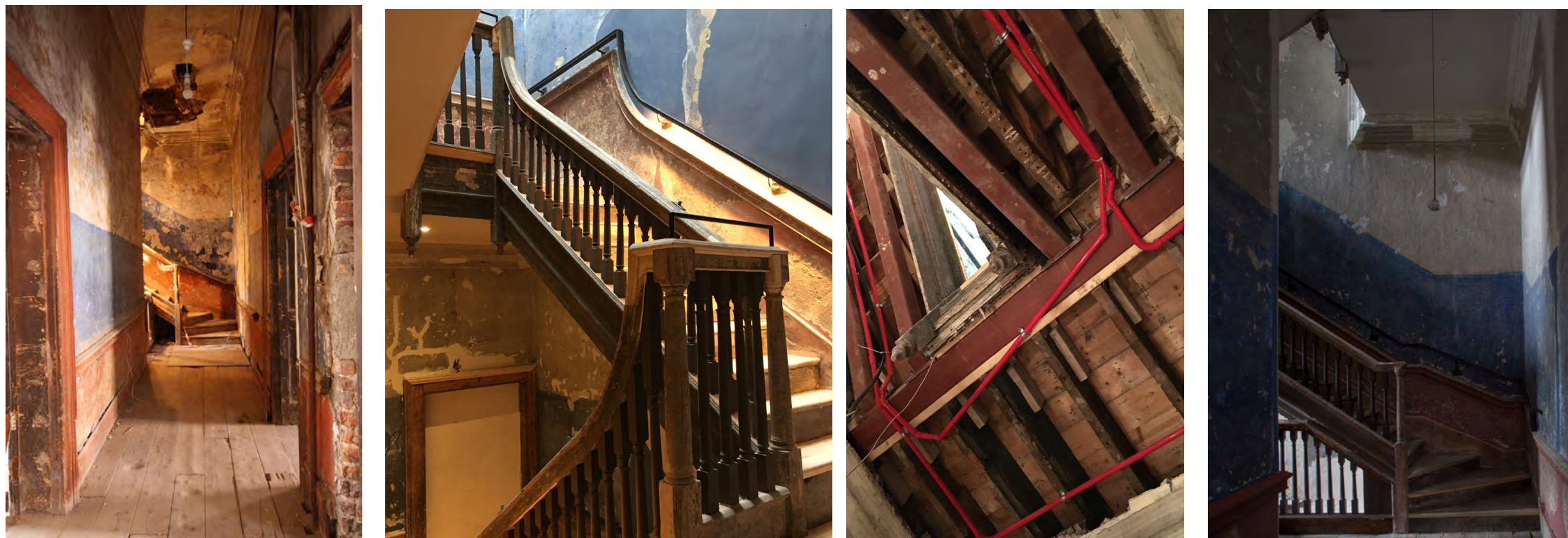
Figs 6.2 to 6.5 (left to right above) illustrate conservation; preservation; restoration and intervention processes within the same space, with fabric before works illustrated at 6.2 and after works at 6.5. In this instance, all processes and associated techniques (repairs; interventions, alterations) are aimed at preserving and presenting historic layers of cultural heritage significance. The interventions indicated in 6.4 have been necessary to meet building regulations.
