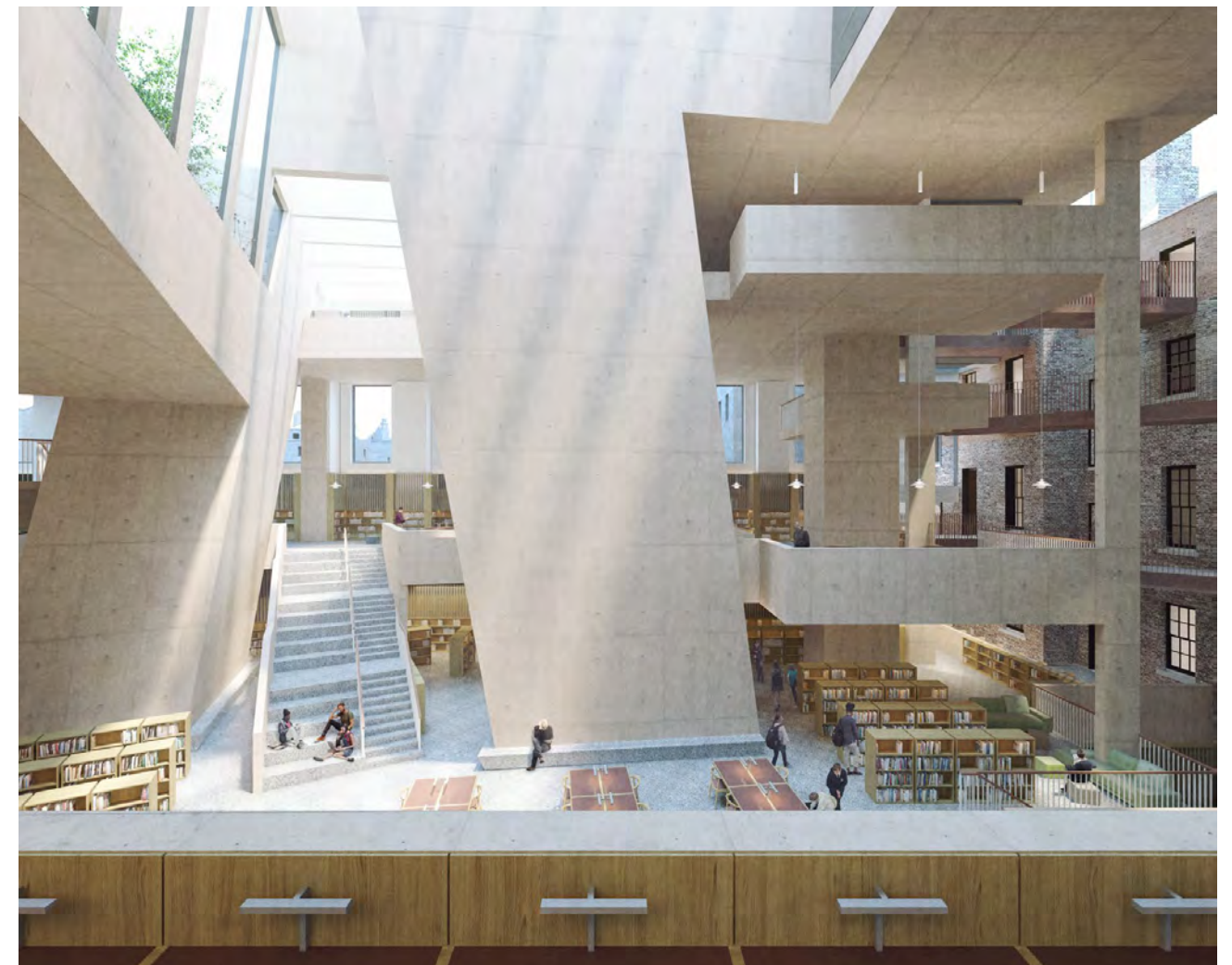
Fig 7.16: View of new build library from first floor/mezzanine level looking east and showing high, rooflit central volume and rear facades of the Georgian houses with bridge links in concrete/steel
